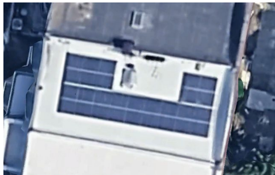
Figure 36: Google Earth Image of Solar Array on the roof of the property.
