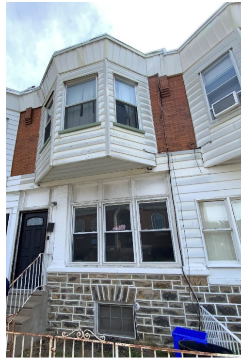
Figure 8: A 2nd floor bump out and framed in porch. Areas with white siding likely hide wood framed walls.
