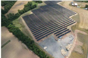
A solar array under construction in 2023 on farmland in Adams County, Pa., that now produces power for Philadelphia-owned buildings, including City Hall. Philadelphia International Report Co. — Reuters Energy
