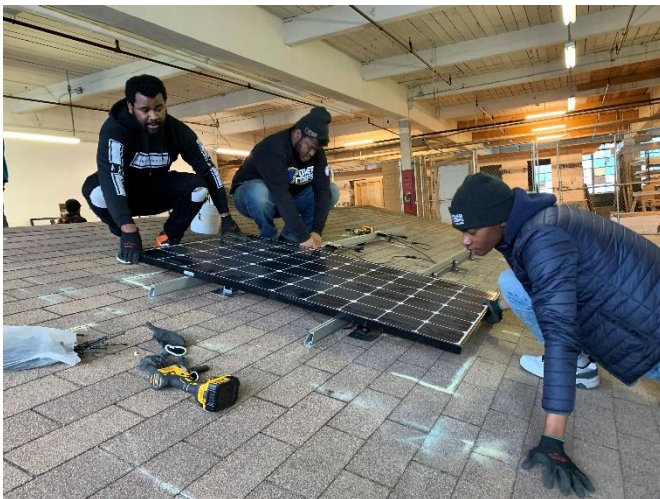
PowerCorpsPHL Solar Fellows practice installing solar. (Credit: PowerCorpsPHL)
