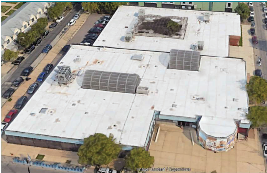
Figure 1. Health Center #5 rooftop.
