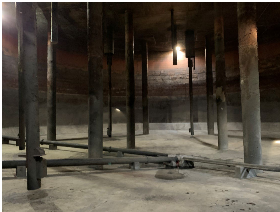
Figure 1: Inside of NEWPCP Digester No. 9
